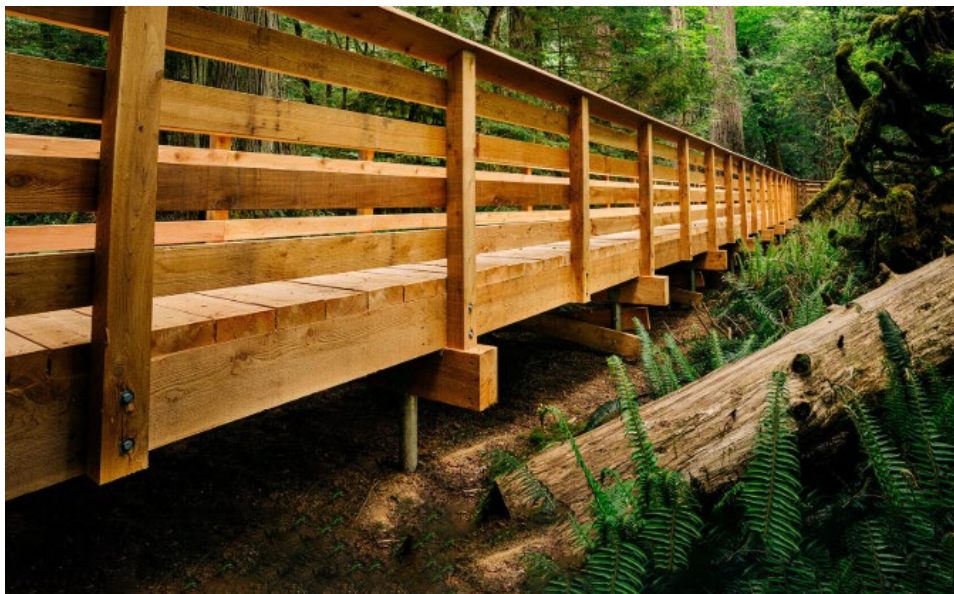
Figure 1: Typical construction for raised wooden boardwalk across wetland crossing.
